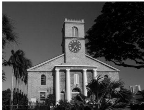
Name: Kawaiahao church Material: Coral rock Founded: between 1836 and 1842 Repair: Past usage:
