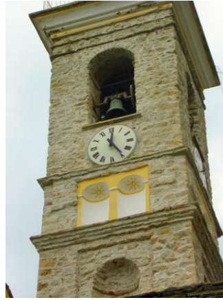
Bell tower or clock tower
