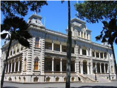
Name: Iolani Palace Material: Founded: Repair: 1969 Past usage: royal palace
